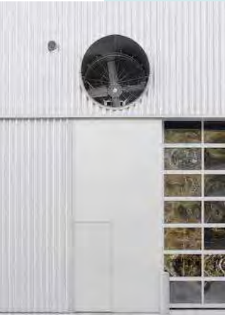
Brandweerkazerne Waterduvel, Mechelen Hub-architects
