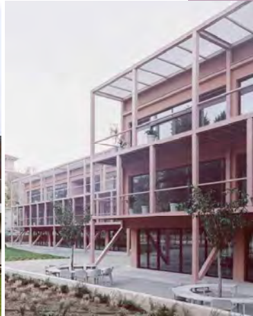
renovatie school Fermi, Tuijn (IT), Bdr bureau
